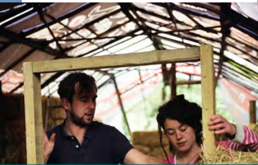
Learn natural building Transition Heathrow, UK
