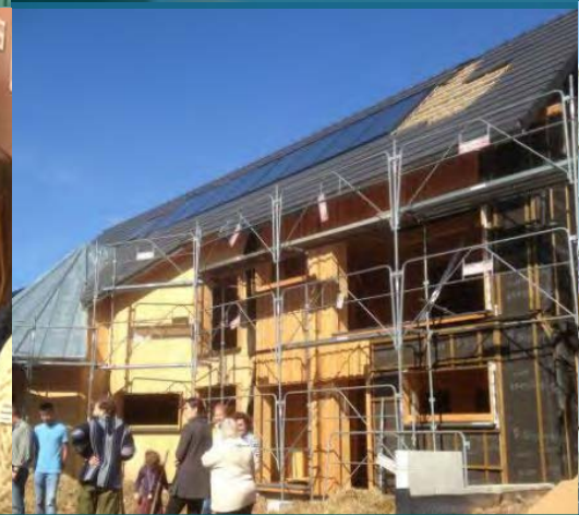
Start a co-housing project Ungersheim, France.
